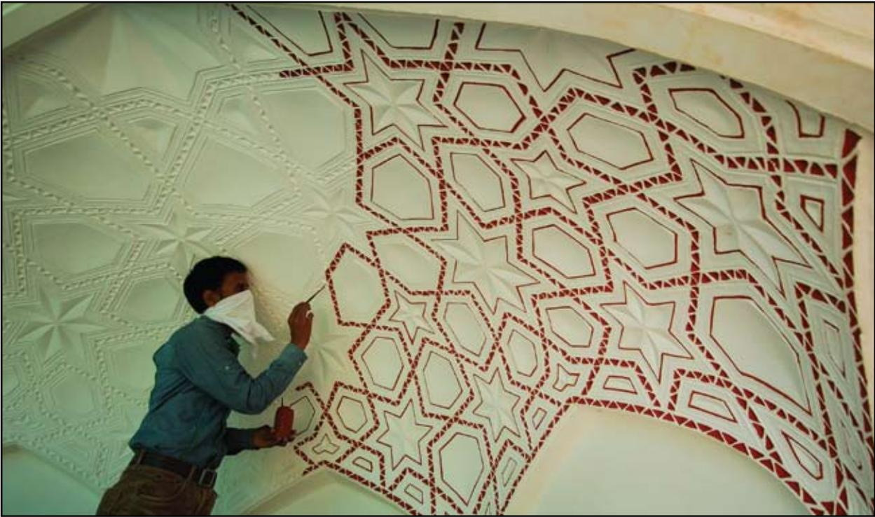
The star shaped patterns adorned the ceilings of the ground level arcade - discovered under cement layers. These patterns were carefully restored on all 68 half-domed arches
