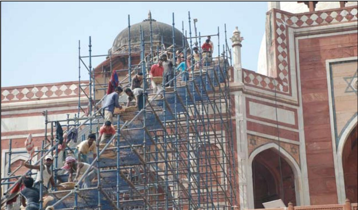
Centuries old building craft traditions were employed in the restoration of Humayun's Tomb wherein modern alterations required to be removed — including 1 million kilos of concrete laid on the roof in the 20th century
