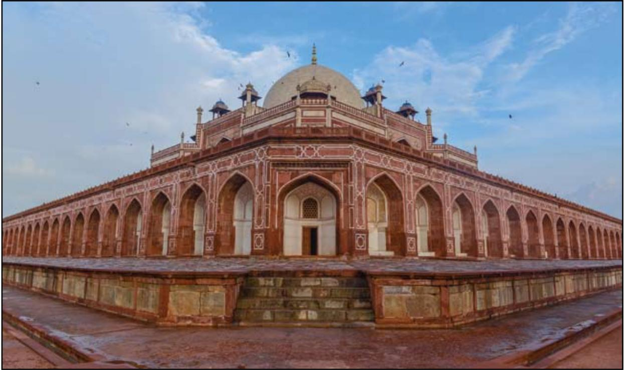
The Humayun's Tomb has a strong diagonal axis with the corners chamfered by the Mughal builders to great effect and canopies marking the corners of the roof
