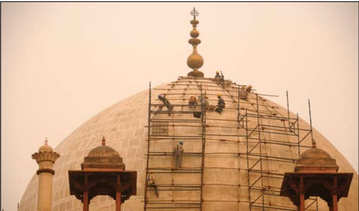
Thousands of stone joints in the dome were required to be carefully filled with traditional lime mortar. The 18 feet tall finial on the dome was also replaced with the original to be displayed at a site museum
